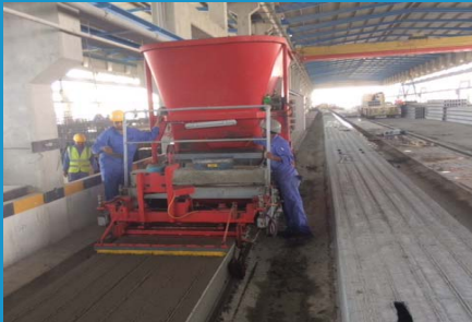
Precast Concrete Area
