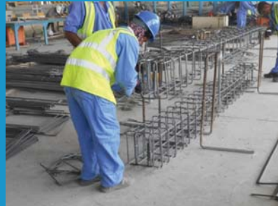
Steel Fixing Area
